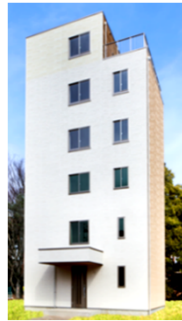
Photo 4 the 6-story 2x4 construction
