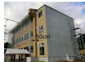
Fire wall (Final test)
